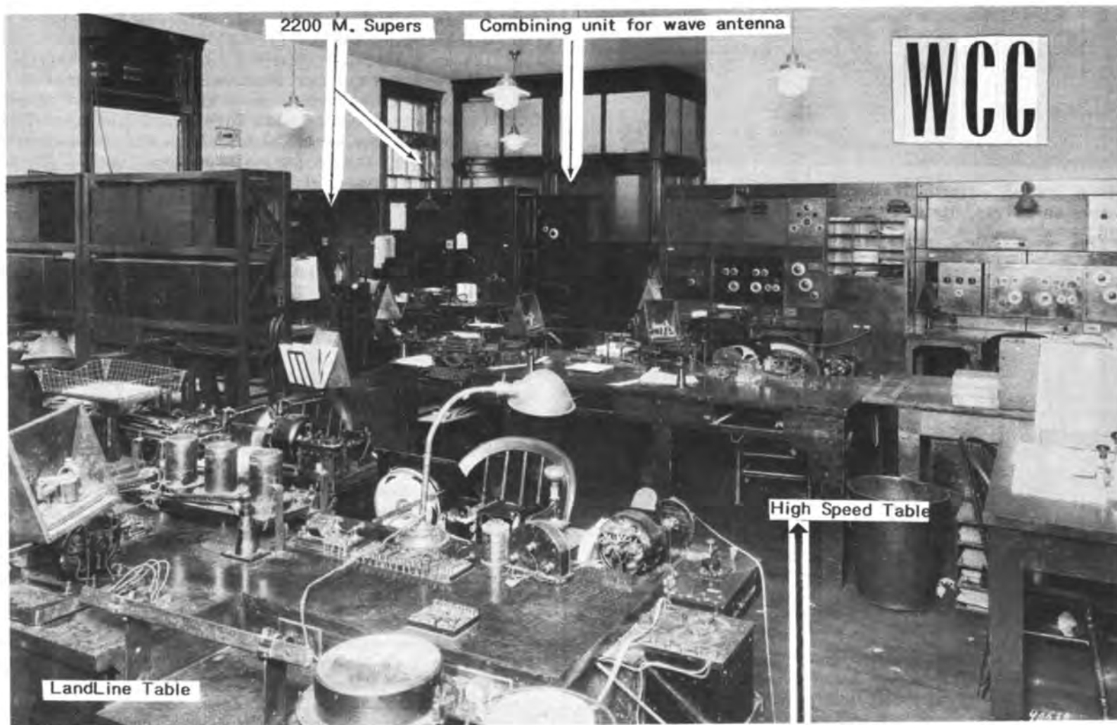
1927 - "WCC", Chatham, Mass. R.C.A. Receiving Station showing station layout with the various components as indicated.
